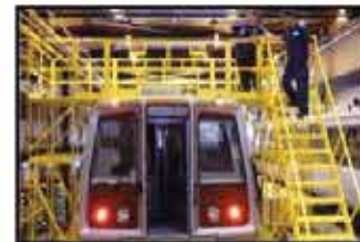
Train Maintenance Platform
