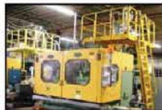
Injection Molding Access Platform
